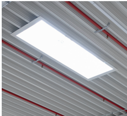
Large skylight domes: for daylight inside the building
