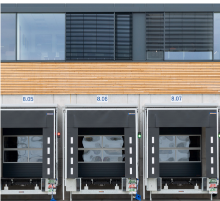
Loadhouses and bays: made to the latest technical standards
