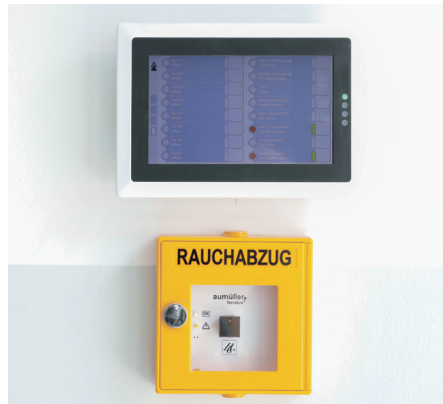
Smart building technology and automatic climate control
