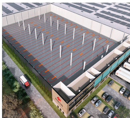
Heating and cooling loops built into the warehouse floor
